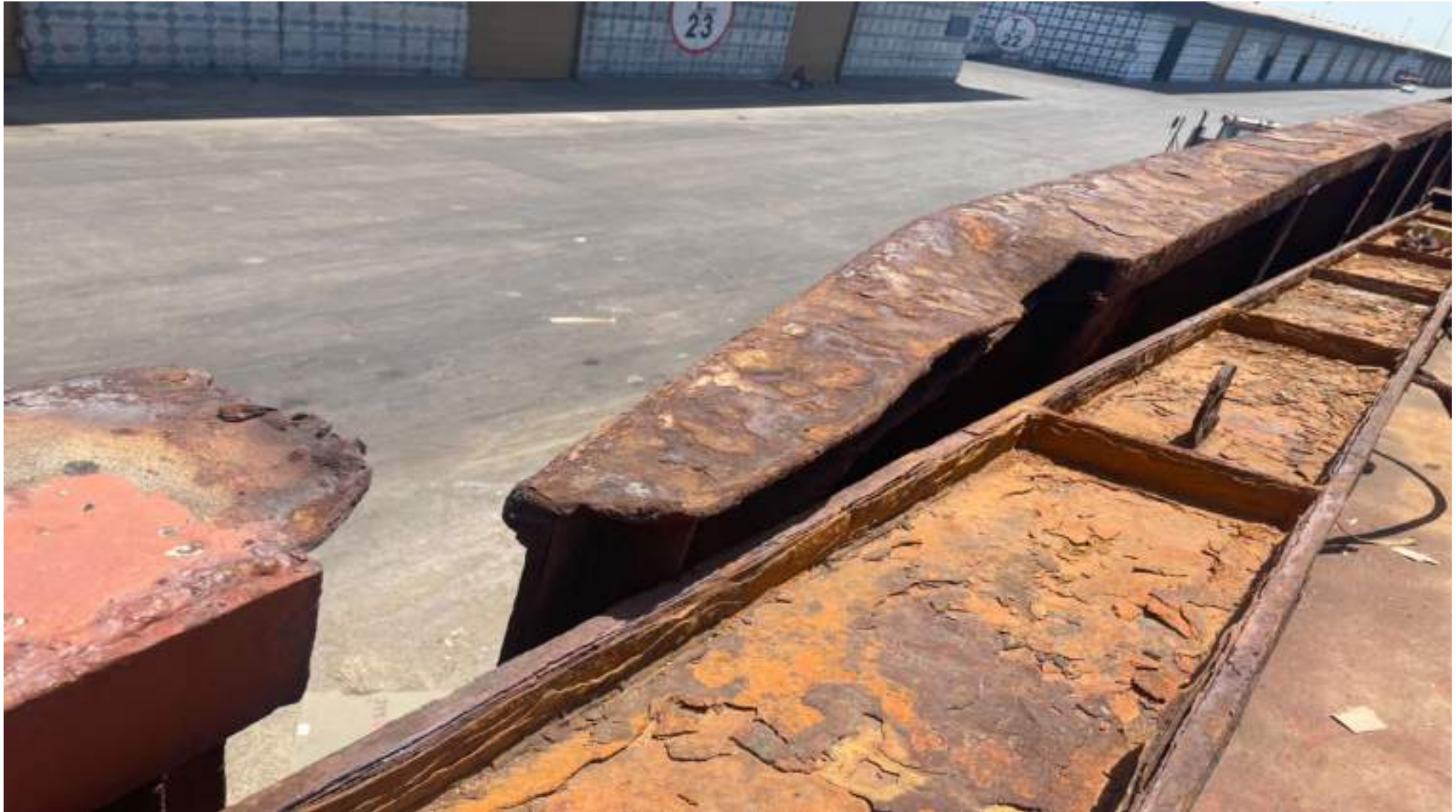
Nature of Deficiency: Decks - corrosion Deficiency Description: Bulwark & guard rails corroded & broken [damaged] PSCO: Mr. Benam Behrouz (Islamic Republic of Iran)
