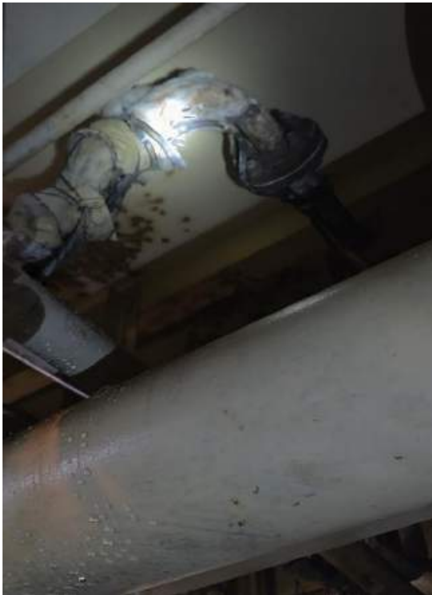
Temporarily fix a leaking ME Jacket cooling pipe
